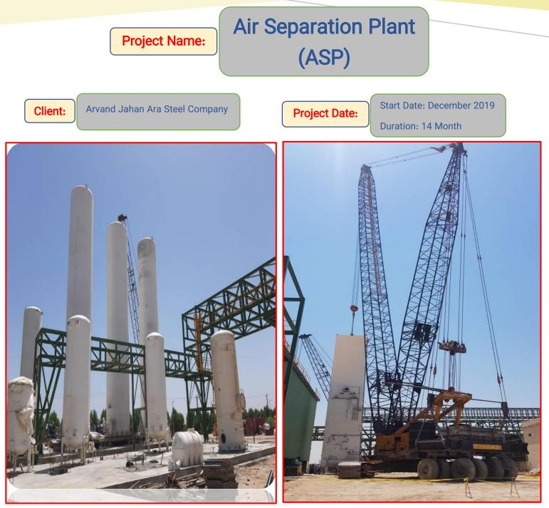
Installation and commissioning operations and cooperation in the commissioning of air separation unit equipments with weight around 810 tons of mechanical equipment installation, 25,000 inches of piping diameter, 24 km of electrical cabling and instruments of the Air Separation Plant (ASP) of Foulad Jahan Ara Arvand Khorramshahr. Designed by SIAD Company in Italy.
