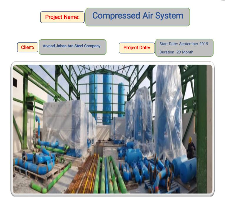
Installation and commissioning operations and cooperation in the commissioning of compressed air station equipment including 80 tons of mechanical equipment installation, 4000 inches of piping diameter, 5 km of electrical cabling and instruments of Compressed Air System Unit (CAS) Jahan Ara Arvand Khoramshahr Steel Company.
