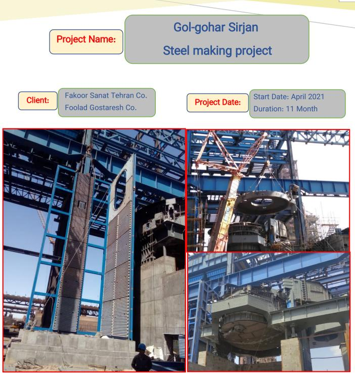
Installation of mechanical equipment of electric arc furnaces and hot rolling furnaces of Gol-Gohar Sirjan steel making project with an approximate weight of 1200 tons. Designed by Sarralle Company in spain.
