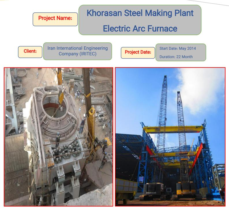
Assembly and installation of mechanical equipment with an approximate weight of 5400 tons and execution of piping lines of about 40000 inches in diameter with all services included in the plans and documents up to the commissioning stage and cold tests of the Khorasan-Neyshabour steel factory. Designed by Tenova Company from Italy.
