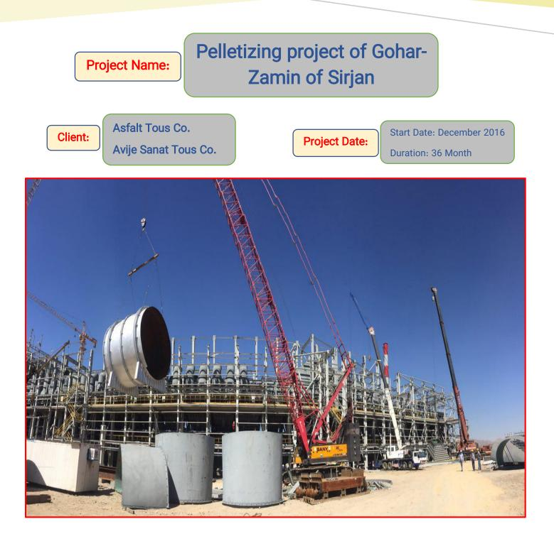
Prefabrication and installation of all mechanical equipment with weight 12,500 tons and implementation of 82,000 inches in diameter along with the pre-commissioning of the Gohar-Zamin pellet factory, Lurgi-Dravo designed by Outotec Company from Germany.
