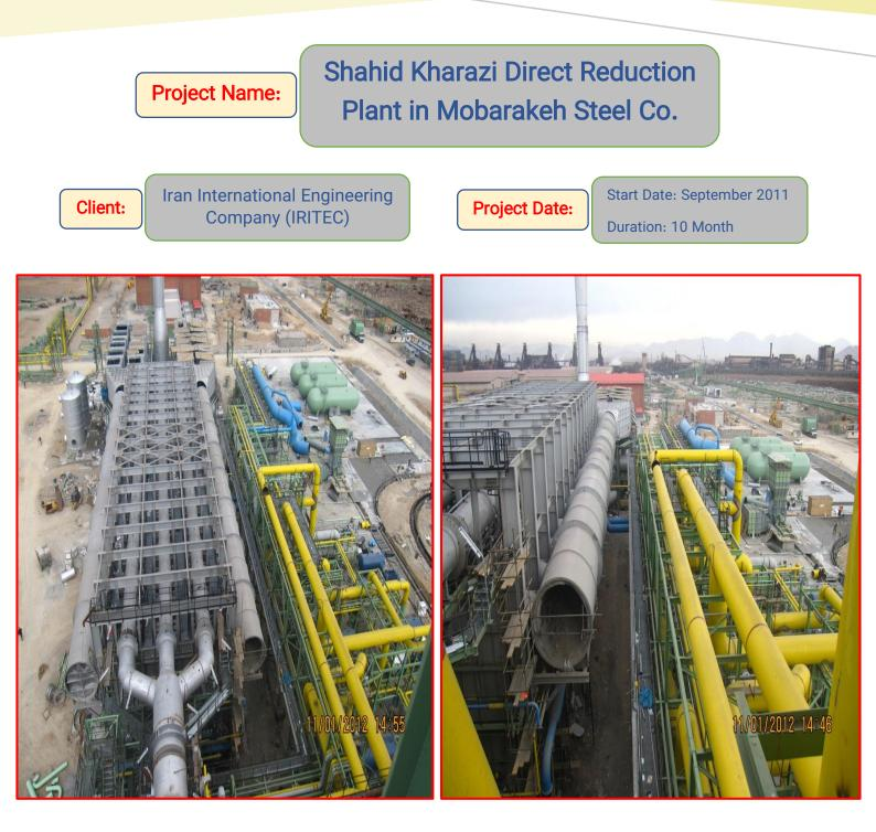
Operation of installation of recuperator ducts and installation of fluid equipment and implementation of piping about 145,000 inches in diameter in Shahid Kharazi direct reduction project of Mobarakeh steel complex in Isfahan.
